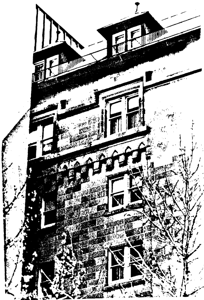
I.1.7.(b) NORTH FACADE - EXISTING ELEMENTS (DETAIL)
