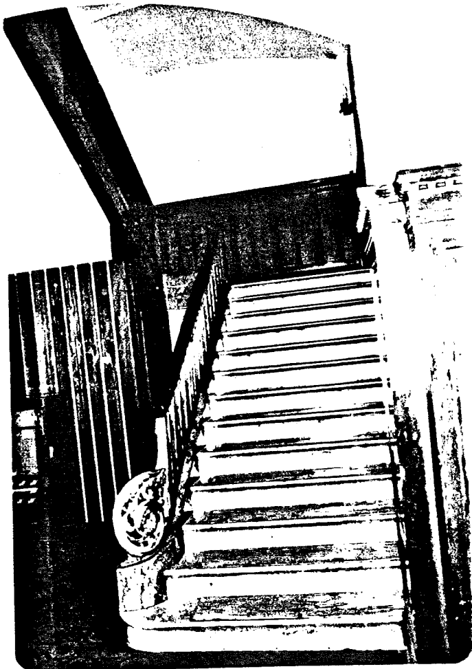
II.1.4.(a) ORIGINAL MAIN STAIRCASE
